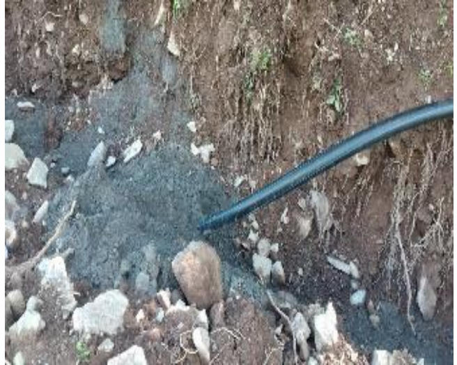
Installation of water supply pipe for Bedoni village
