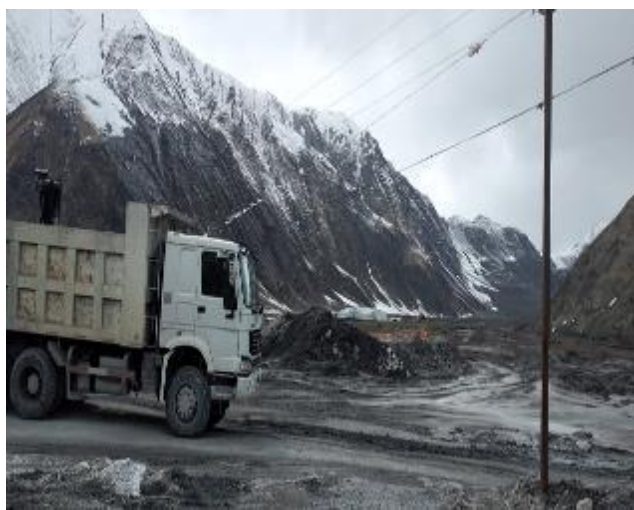
Overhead cable at cruching plant
